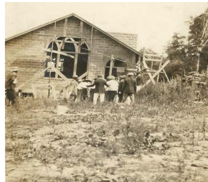
Rebuilding of Ebenezer Baptist Church 1923-24
