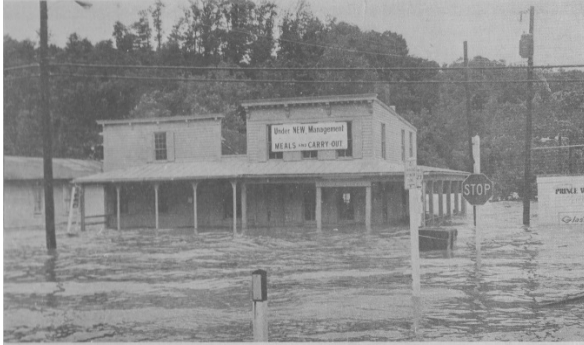
Occoquan Inn 1972- Hurricane Agnes
